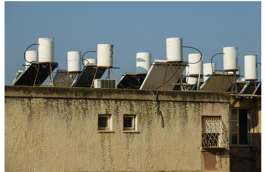
Rooftop solar thermal water heating systems
