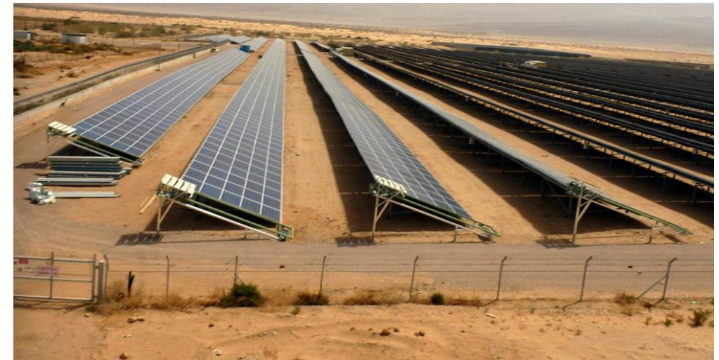
Solar field, Kibbutz Elifaz
