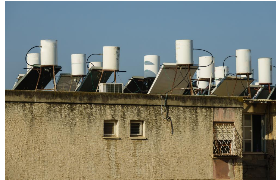
Rooftop solar thermal water heating systems
